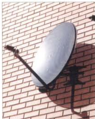
Fig. 1: Off-set fed dish - the dish is 'looking' 25° above the apparent line of sight.
